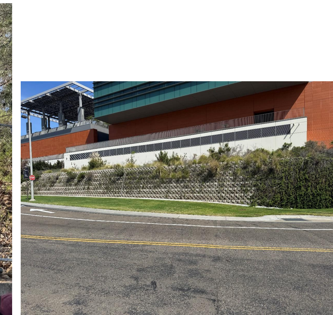
Image 7: Retaining wall below west side of Storm Hall.
