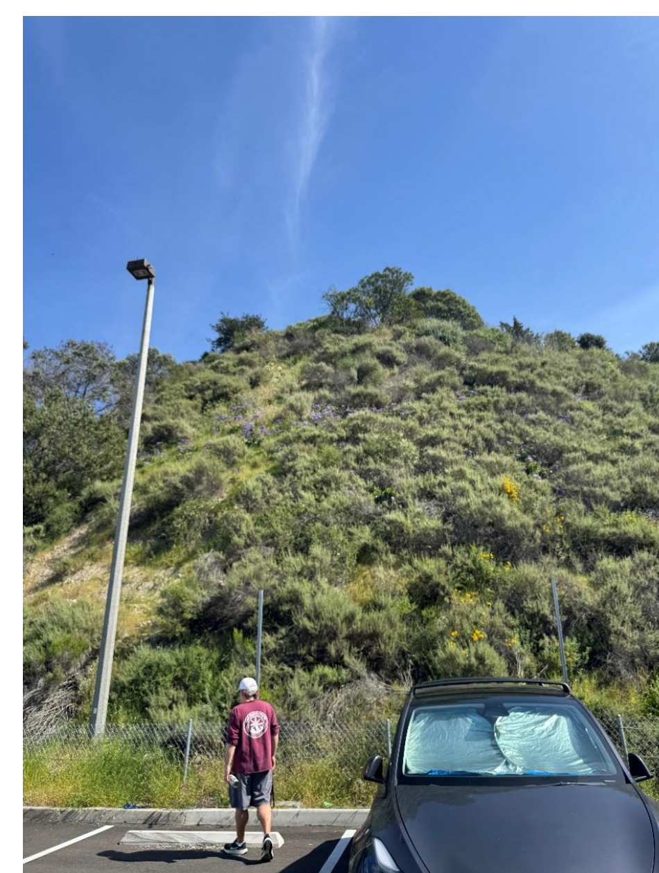
Image 9: ~65° angle of repose on hillslope north of parking structure 14.
